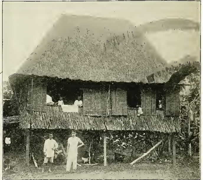
FIG. 202. — A house in the Philippines, built of bamboo and covered with thatch. The house is raised above the ground because of the dampness.
